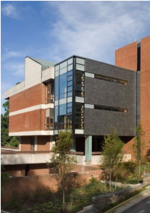
Campbell Hall addition
