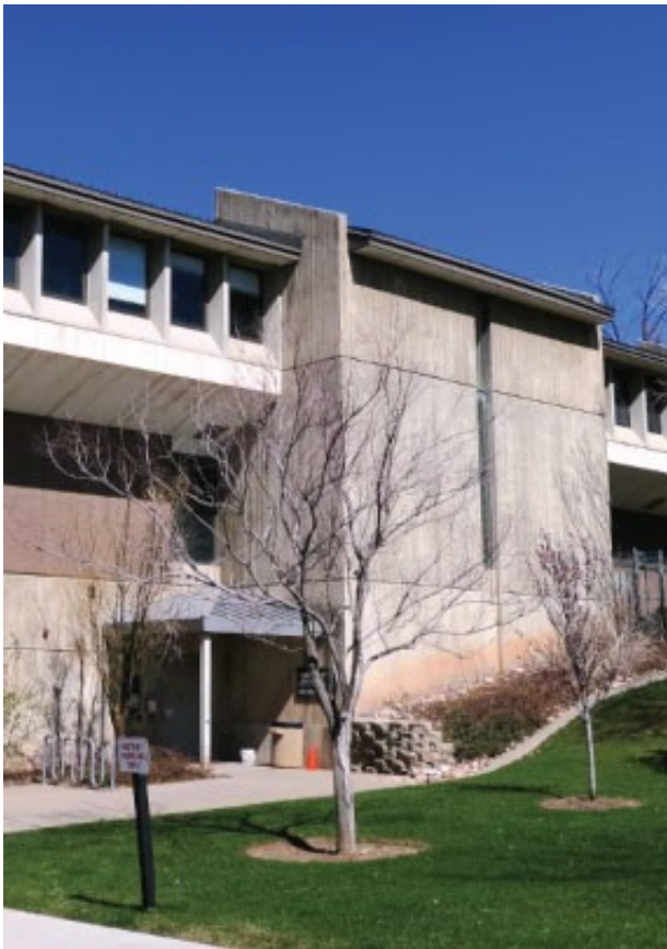
Side view of Dumke Health Building
