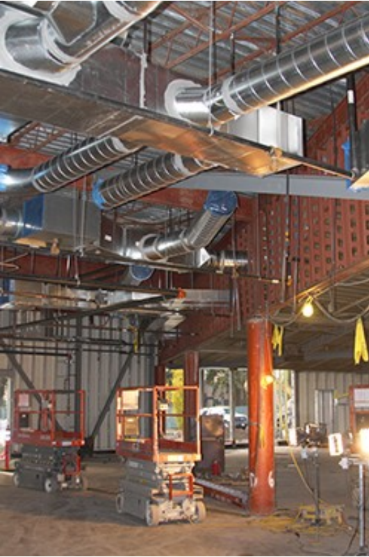
New duct work
