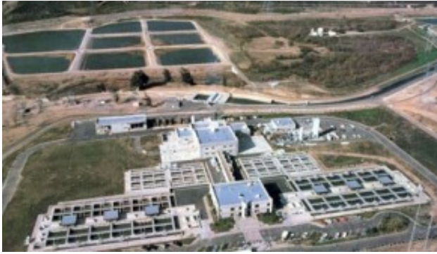
Overhead the Los Angeles Aqueduct Filtration Plant
