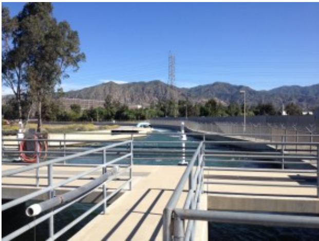
Los Angeles Aqueduct Filtration Plant headworks
