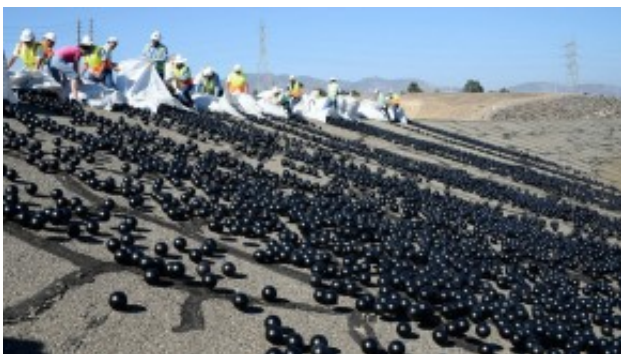
Shade balls being used to cover the reservoir
