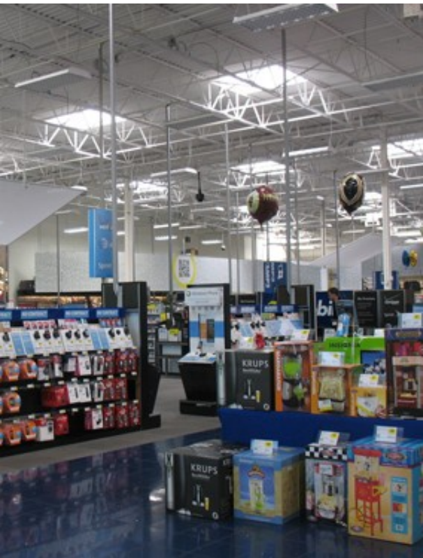
Skylights with dimmable fluorescent lighting
