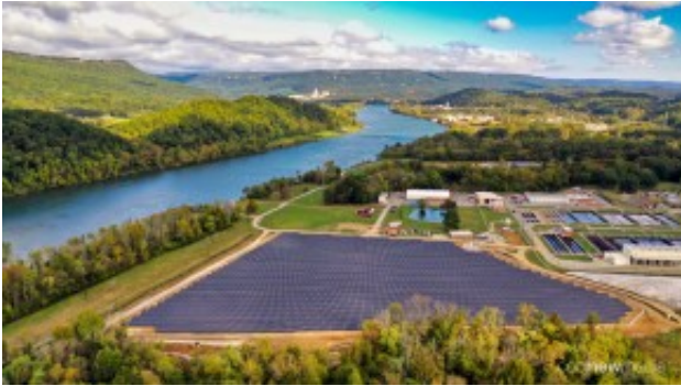
Moccasin Bend Environmental Campus Solar Panels
