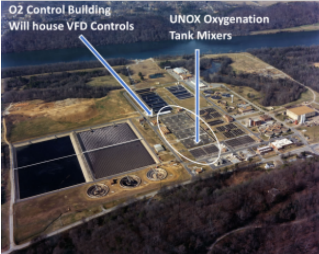
Moccasin Bend Environmental Campus VFD
