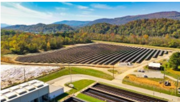
Moccasin Bend Environmental Campus Solar Panels
