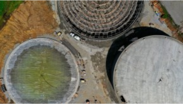
Moccasin Bend Environmental Campus EQ Station Exterior
