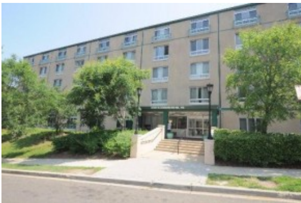
Front Façade of Fort Lincoln
