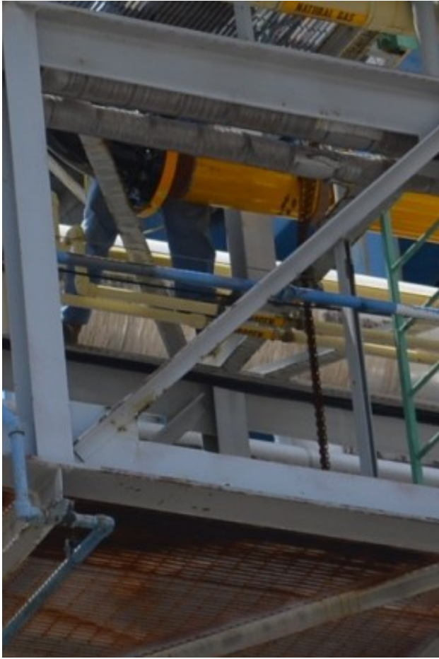
New Natural Gas header (dark yellow)
