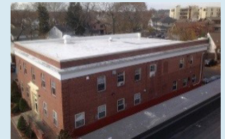
The public shelter, Operation Hope Fairfield, will be energized 24/7 because of the microgrid. Photo courtesy of Schneider Electric.
