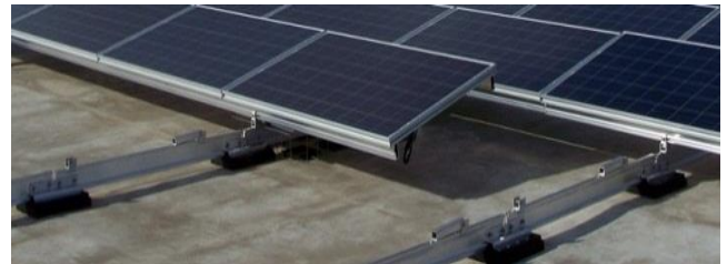
Attached PV Racking System Photo credit: SunLink
